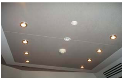
Fig 1. Serenity Ceiling Panels can be designed to fit around existing services, or even incorporate new services, such as lighting.
